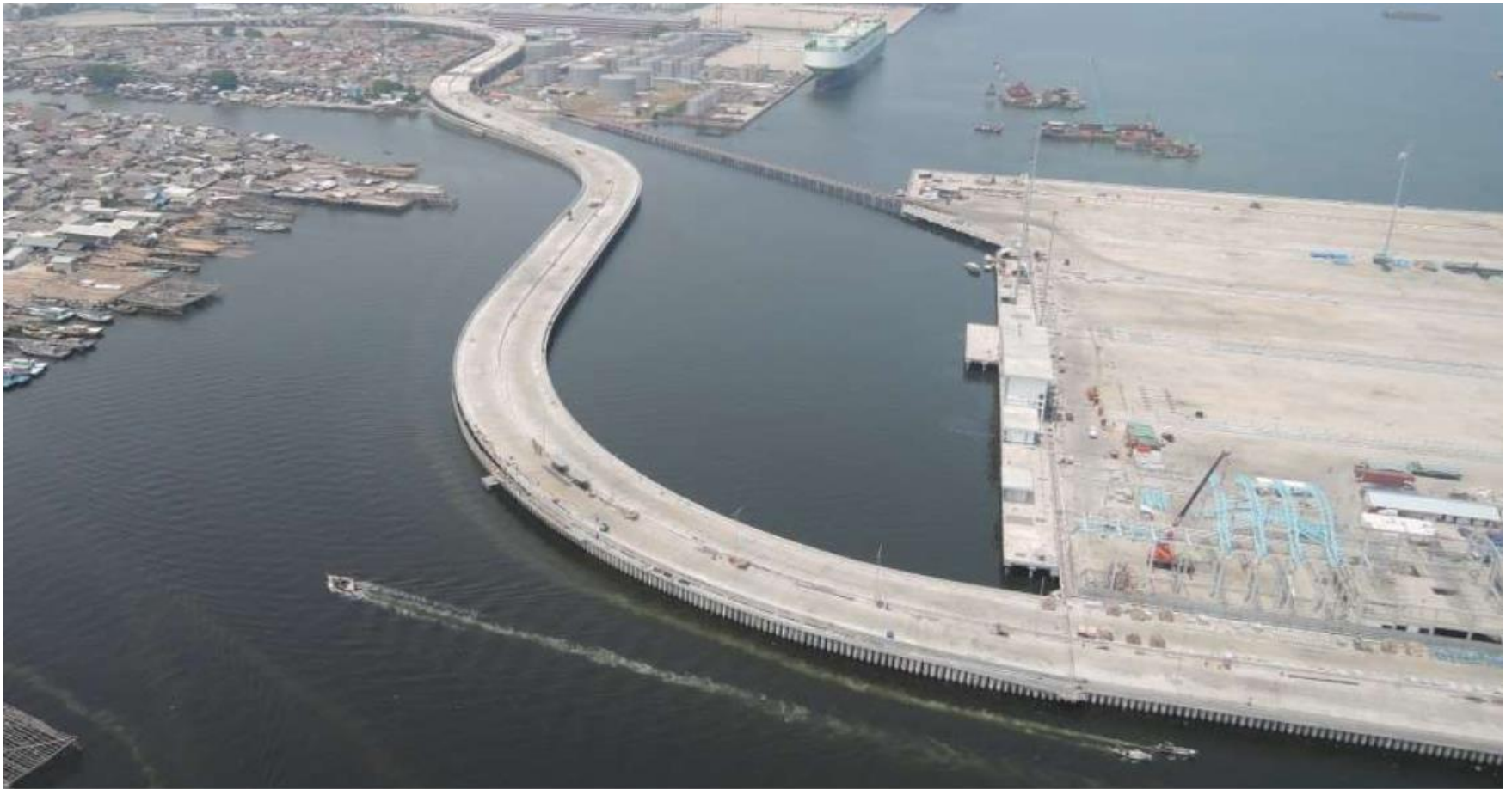
Access Road (Sea Side) - 700 m of length
