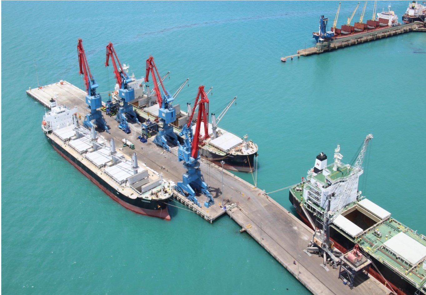
4 units Gantry Luffing Crane
